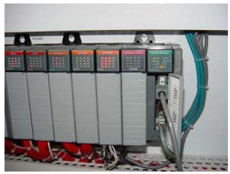
With each module having sixteen "points" of either input or output, this PLC has the ability to monitor and control dozens of devices. Fit into a control cabinet, a PLC takes up little room, especially considering the equivalent space that would be needed by electromechanical relays to perform the same functions:
